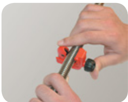
1. Measuring and cutting the hose
